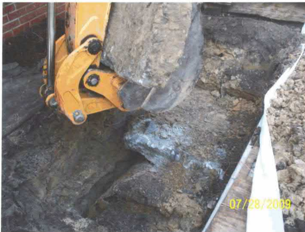
Picture 2: UST 1400Eagle removal operation.
